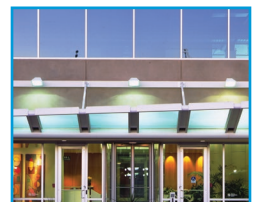
outdoor facility lighting
